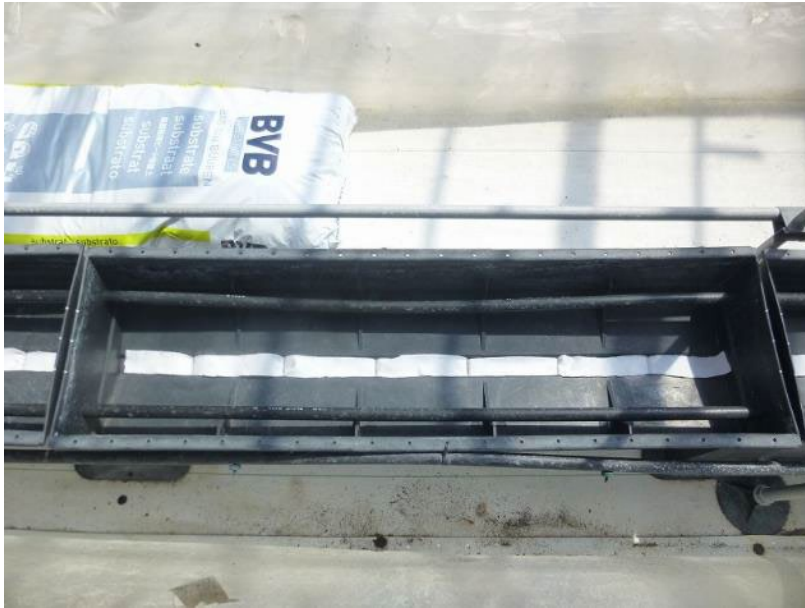
Growing bed before filling with medium. The fabric outside of the drainage opening improves drainage.
