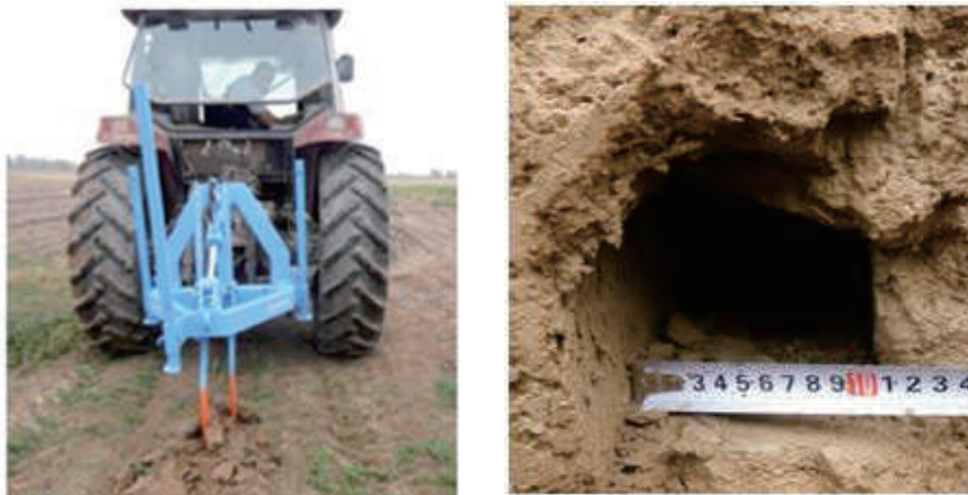
Fig. 6 Drilling situation of the Cut drain operated in Uzbekistan
