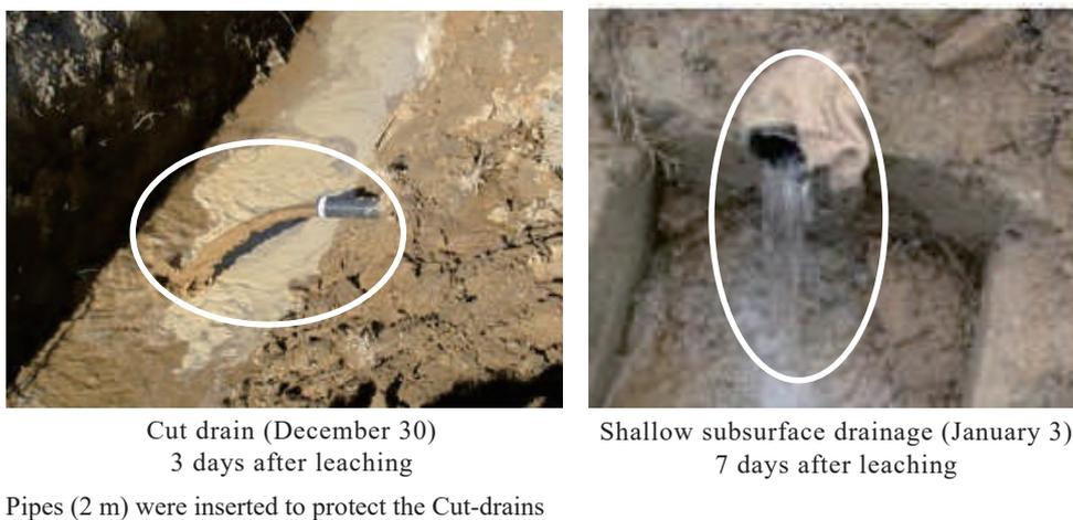
**Fig. 7** State of discharging from outlets after leaching
