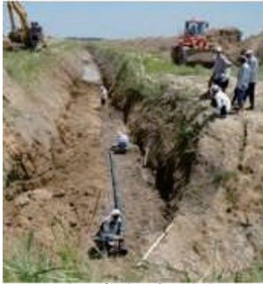
Construction of subsurface drainage
