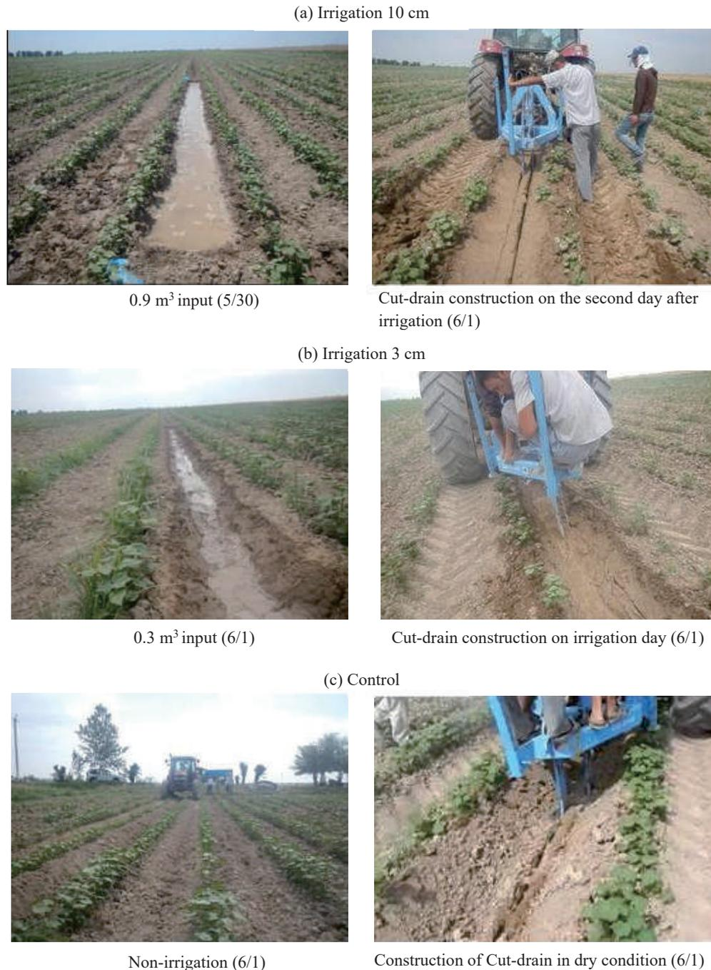
**Fig. 6** Cut-drain construction under different irrigation conditions
